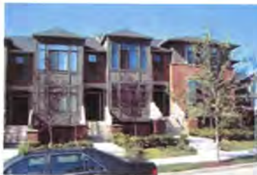
These townhomes use brick, decorative windows and a decorative entry design.
