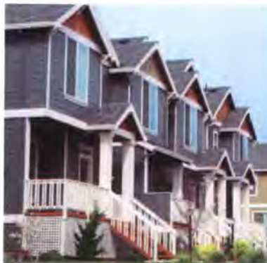
Workforce housing may take the form of single family detached or attached homes or units within mixed use or residential buildings.
