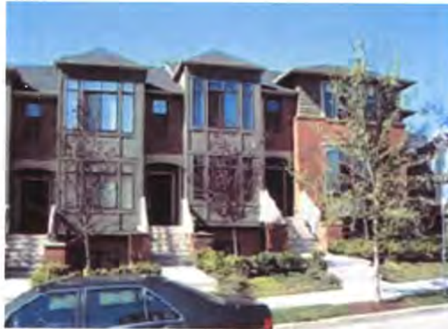
These townhomes use brick, decorative windows and a decorative entry design.
