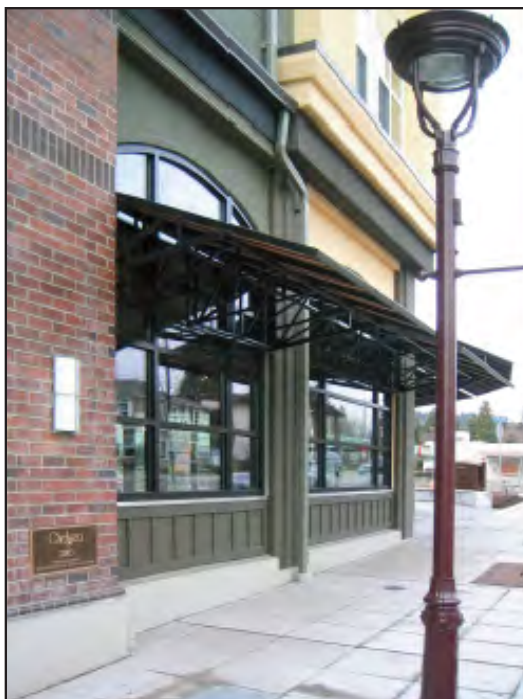
This building uses lighting, decorative materials, a canopy and windows.
