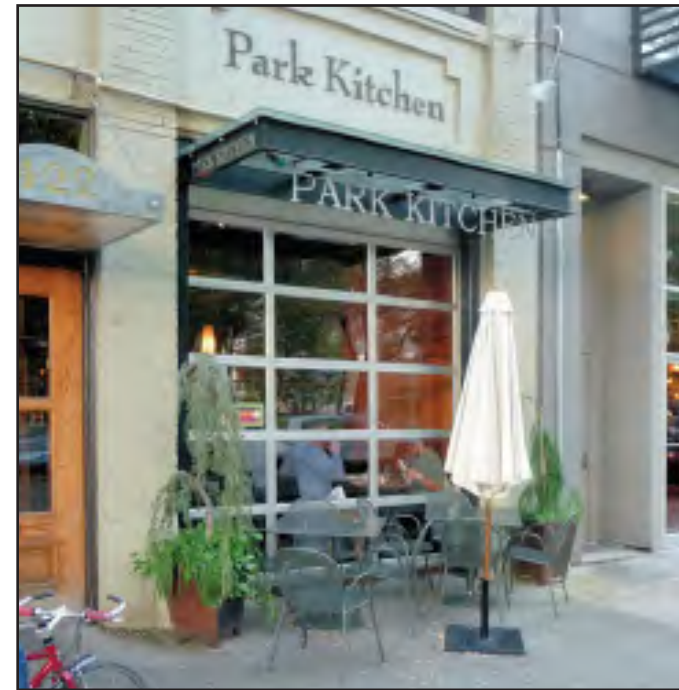
This façade uses a roll-up door, steel canopy and decorative lighting.
