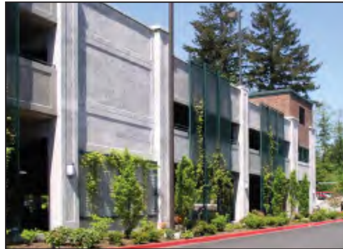
This parking structure is masked with decorative plantings and trellises.
