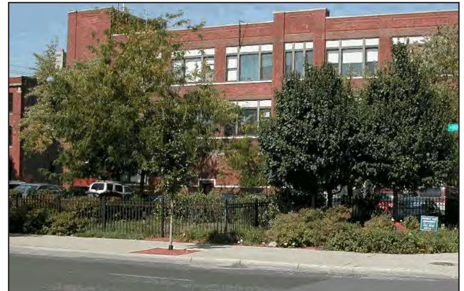
A decorative low wall and landscaping conceal parking from the street.
