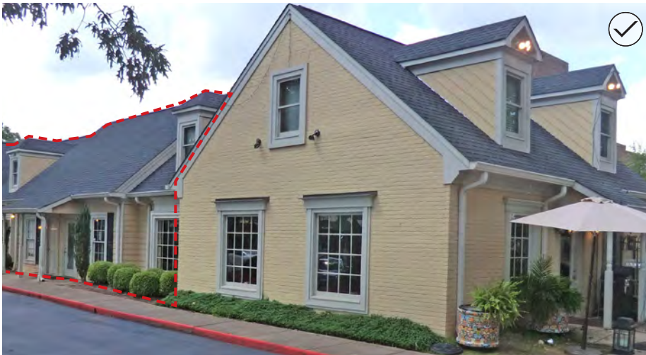
Design an addition to be compatible with the scale, massing and rhythm of the historic context.
