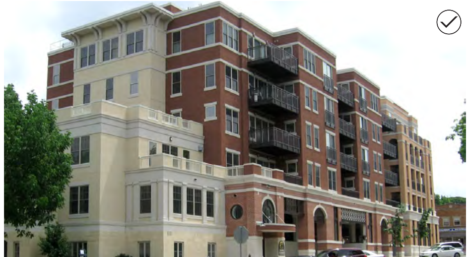
Use moldings, columns, a change in material, or offset in the wall plane to define vertical modules.
