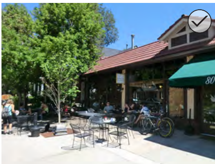
Locate buildings to create well-defined street frontages and promote active, pedestrian-oriented streets.
