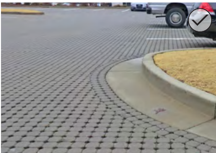
Reducing paved areas (top) and installing permeable paving systems, such as the pavers used in the parking lot at 11261 Alpharetta Highway (bottom), allow rain water to percolate into the ground underneath.
