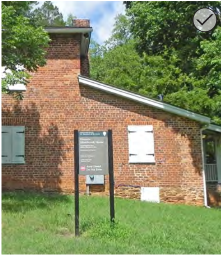
Preserve the original roof form of a historic structure.
