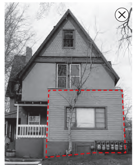
Do not locate an addition in front of, or flush with the primary façade.
