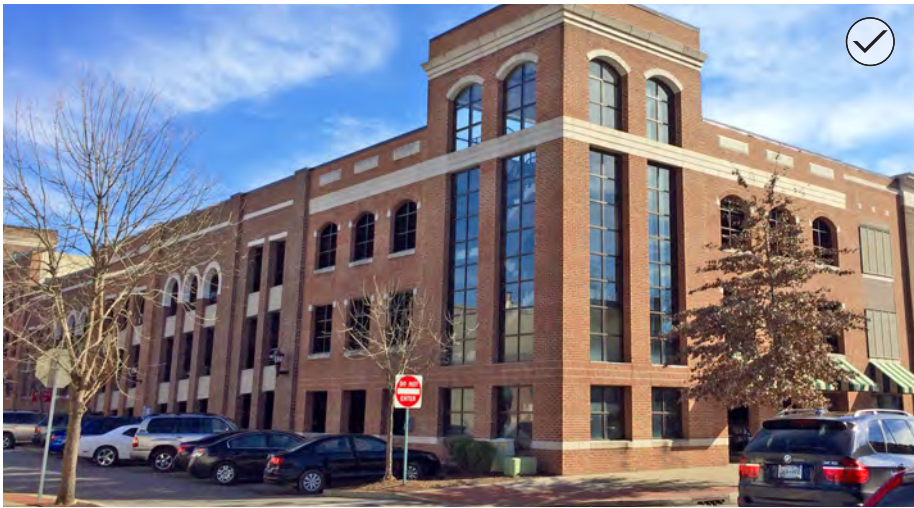
Divide a larger parking structure into modules that reflect traditional façade and lot widths in the historic district.
