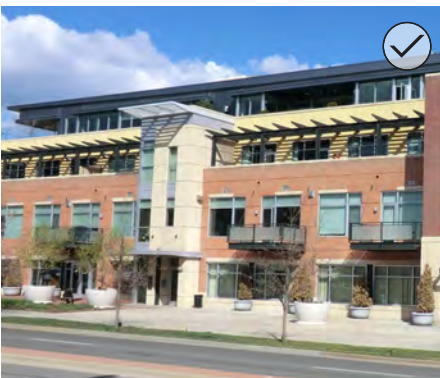
Set back a larger building mass from the street wall when possible to reduce looming effects.
