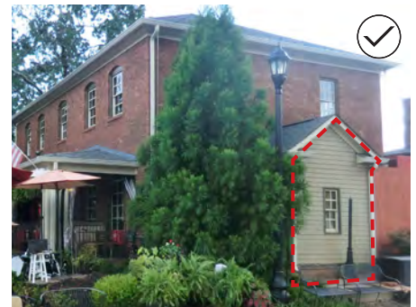
Locate an addition to a historic structure to be subordinate to the primary building.
