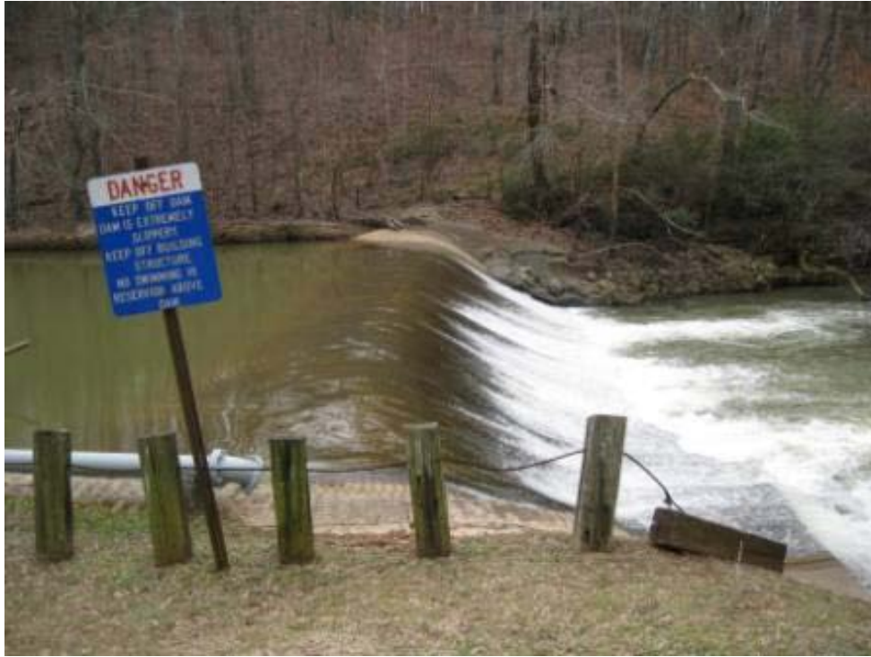
Figure 9 - View of Big Creek along Oxbo Road.
