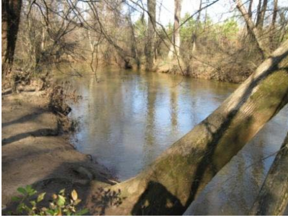
Figure 3 - View of streambank erosion on Big Creek.
