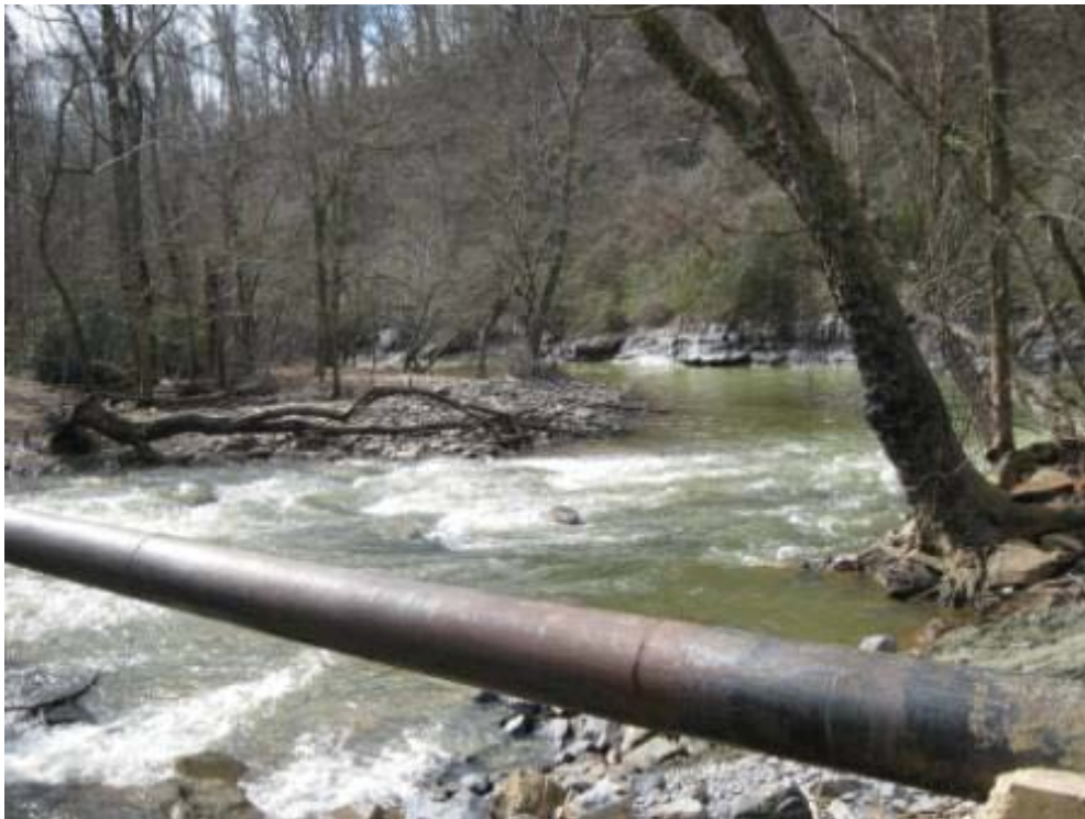
Figure 10 - View of sewer crossing near Roswell Mill.
