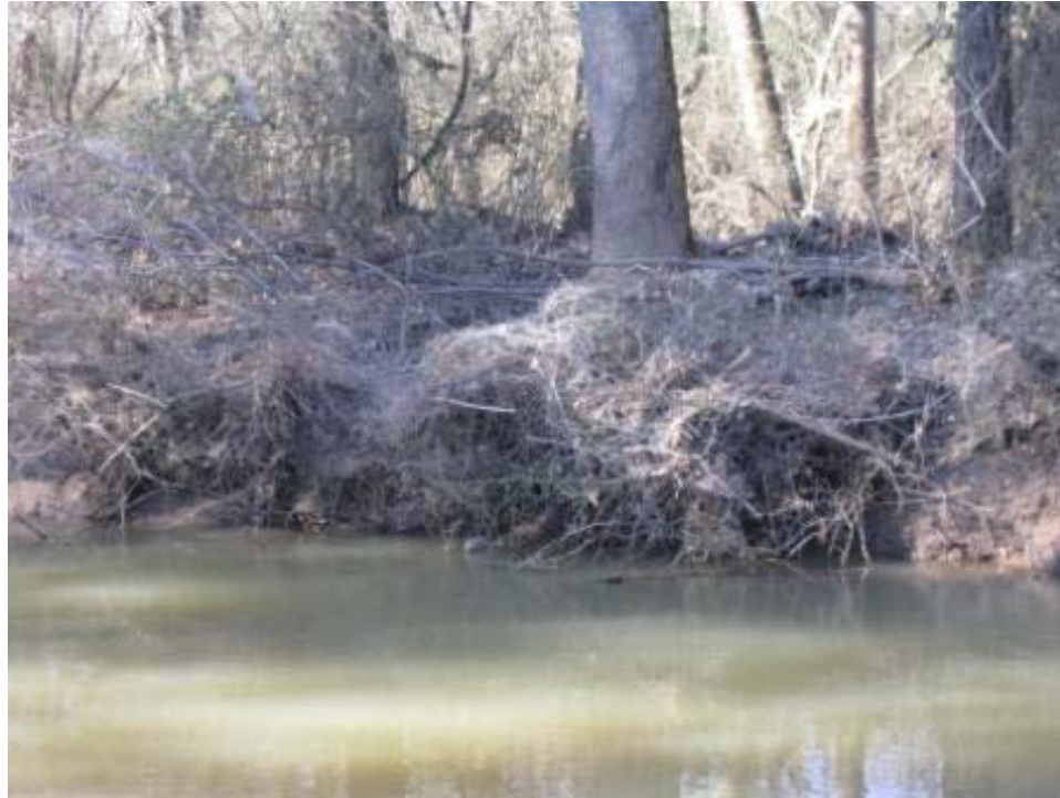
Figure 5 - View of localized streambank erosion.
