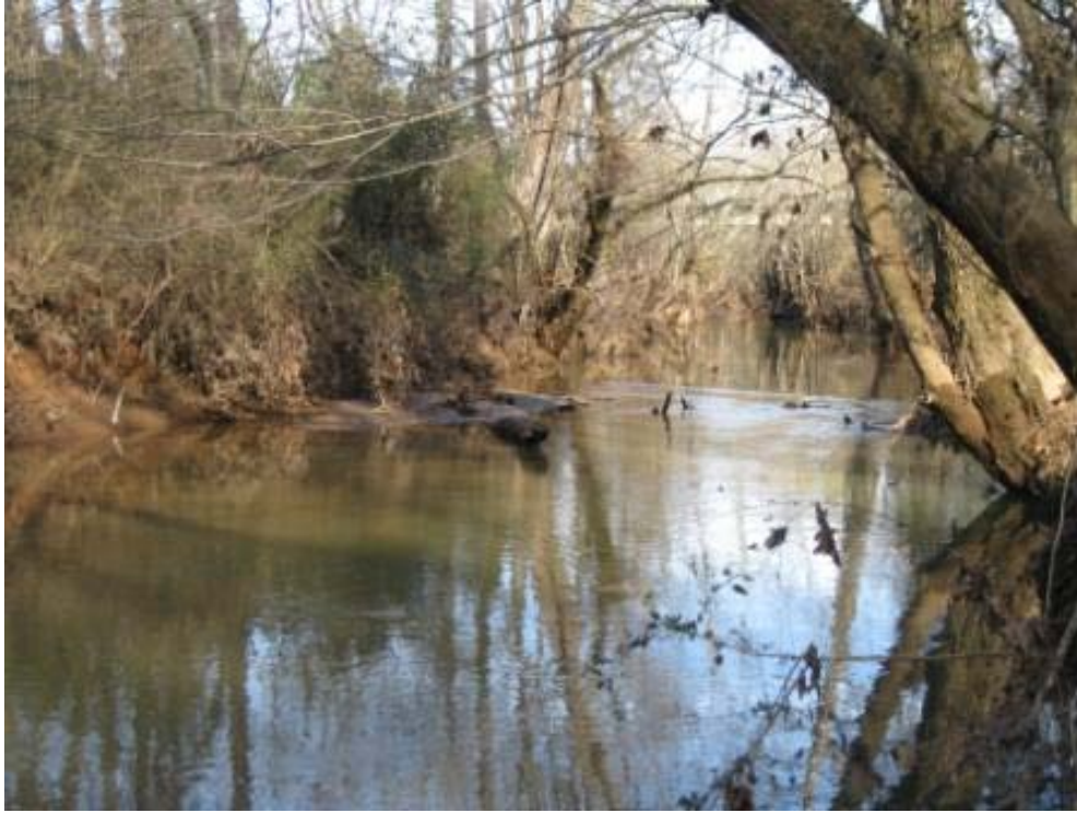
Figure 9 - View of stream bank scour near Davis Drive.
