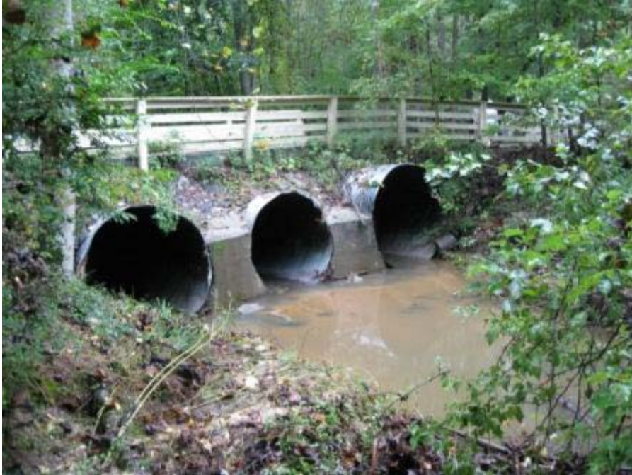
Figure 1 - View of culvert at Roswell Area Park
