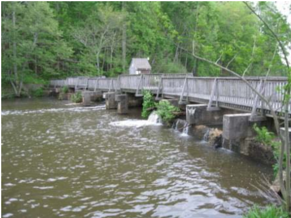
Figure 10 - View of spillway from Garrett Lake.
