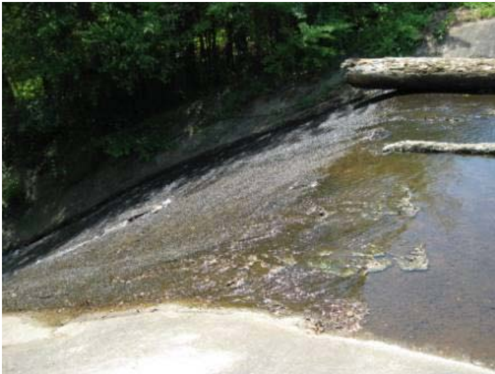
Figure 6 - Spillway on East Spring Lake on tributary to Willeo Creek.
