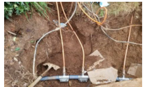
Photo of GS Line Being Replaced in a Cul-De-Sac
