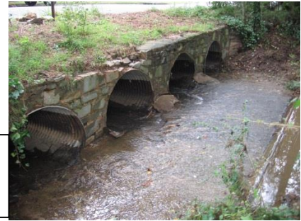
Photograph 2: Worthington Hills Drive culverts maintained.
