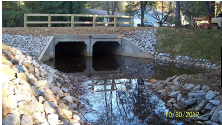
Photograph 3: Worthington Hills Drive culverts replaced.
