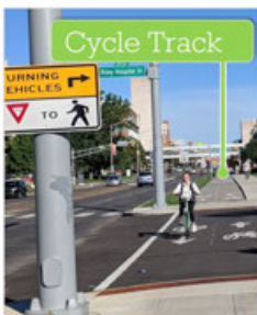
Cycle Tracks – An area delineated for bicycle travel physically separated (through raised pavement or a large striped area) from the vehicular roadway
