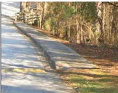
Hazardous surfaces, lack of curbs and buffers, and “sidewalks to nowhere” are common conditions for pedestrians.
