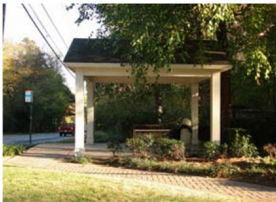
Bus shelter at Chattahoochee Landing apartment complex
