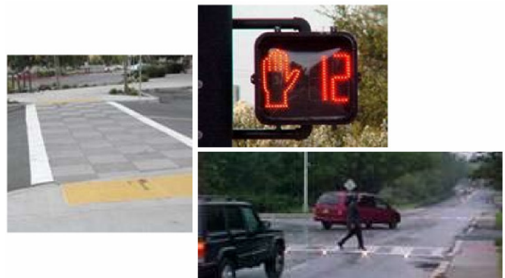
Implementing a range of traffic calming strategies, such as textured pavement, countdown signals, and in-pavement lighting, will make the Town Square safer and more welcoming for pedestrians.
