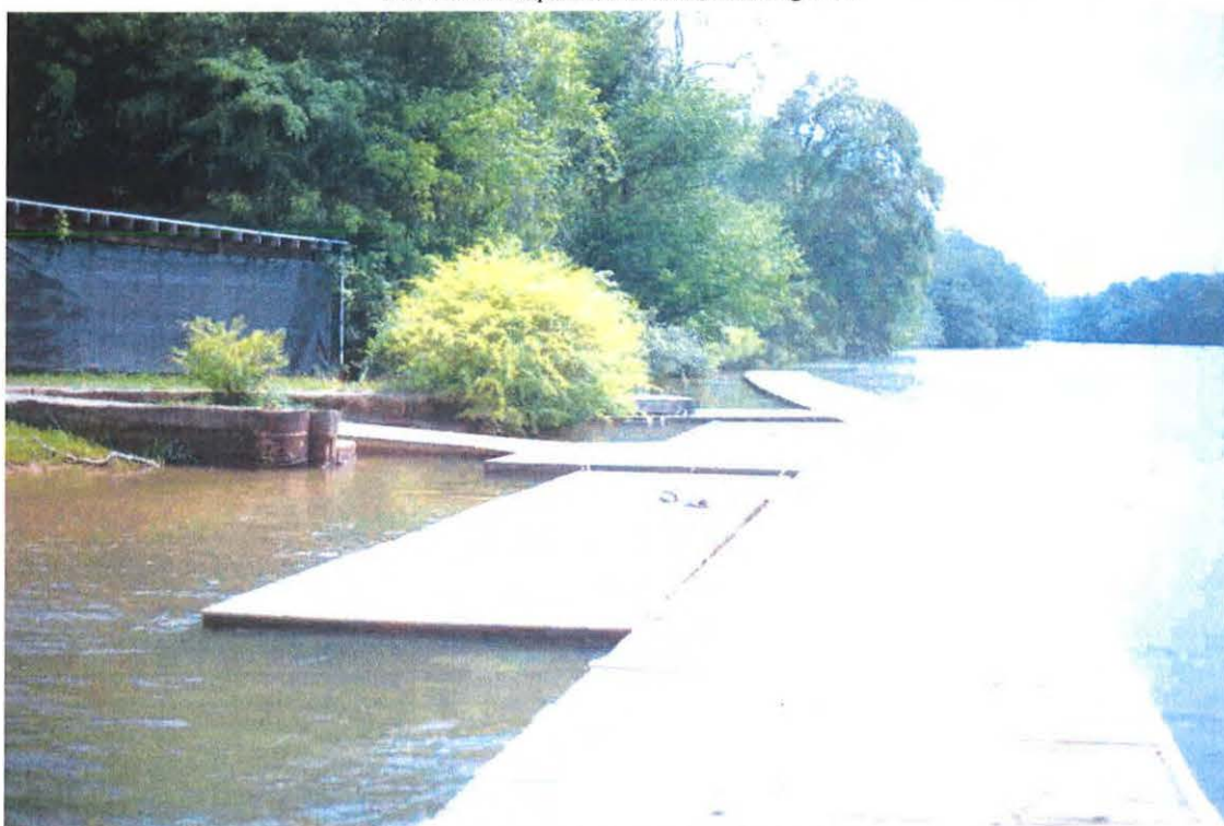
Site of the Existing Boat Dock, Looking Northeast
